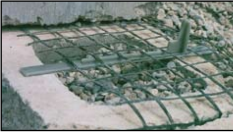
Earthworks block retainer placement during construction.
